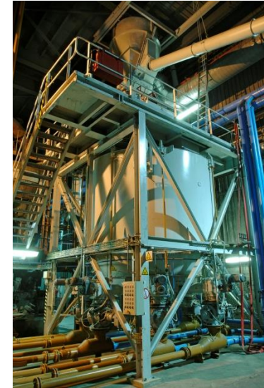
T4 Grinding mills
